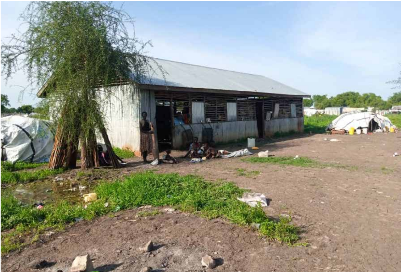
Figure 3. IDPs in Pibor have been displaced to a local school building (2020)
