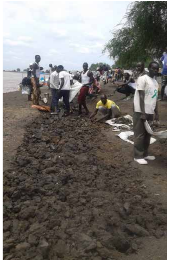
Figure 18. Community volunteers build a new dyke in Jikmir, Nasir
